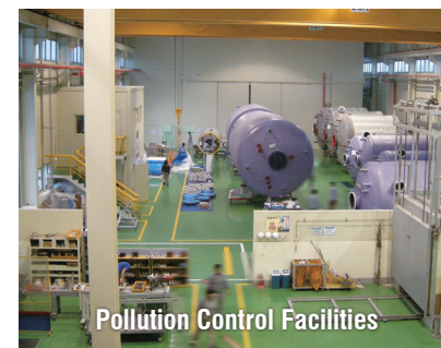
WWT, DI, UPW System
